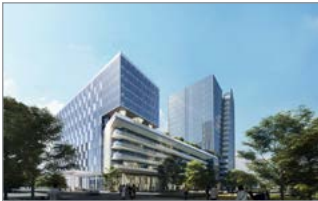
THE TOWER AT HALL PARK Far North Dallas 386,946 RBA 386,946 Max Contig. SF Withheld Rents Hall Group
