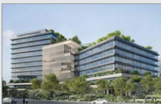
GOLDMAN SACHS Uptown/Turtle Creek 702,000 RBA Lease signed Build-to-Suit Breaking Ground 10/23 Hunt Consolidated
