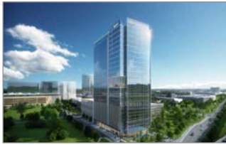
RYAN TOWER Far North Dallas 409,182 RBA 205,004 Max Contig. SF Withheld Rents Ryan Companies
