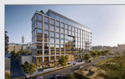
CRESCENT OFFICES WEST South Fort Worth 170,000 RBA 170,000 Max Avail. SF Withheld rents Crescent Real Estate
